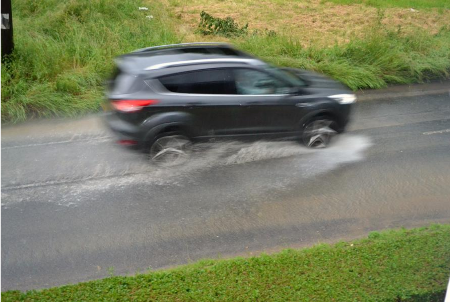
Figure 3 Flooding in Bull Lane
